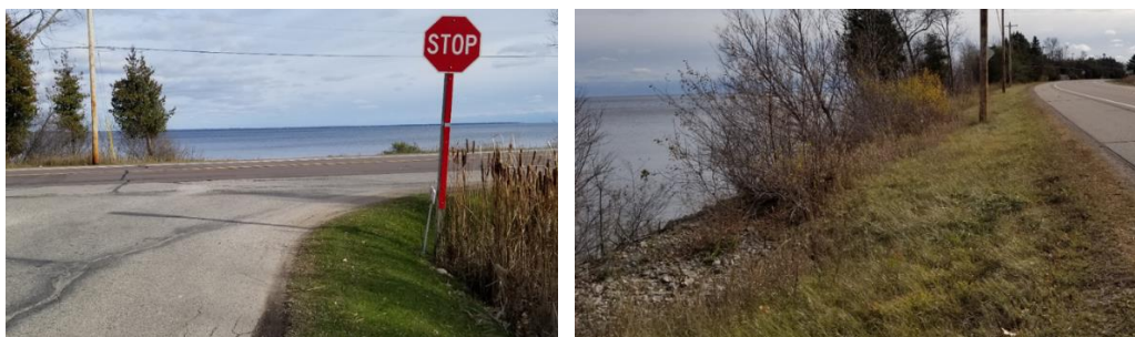
Figure 14: Infinity Effect (left) and Roadside Slope (right)
