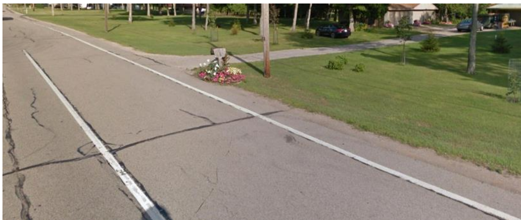
Figure 16: Passing Flare at Airport Road
