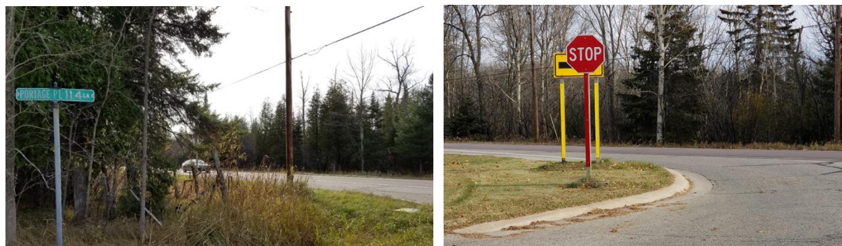
Figure 15: Limited Sight Distance (left) and Conflicting Signs (right)
